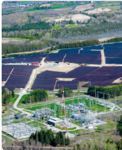
UTILITY ASSET MANAGEMENT WITH AURORA VISION IN PARALLEL WITH SCADA SYSTEMS
